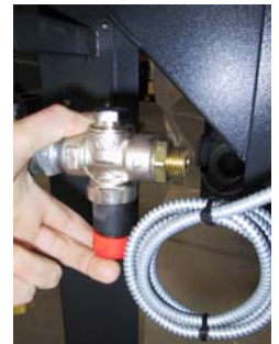
Sprinkler valve without hose
