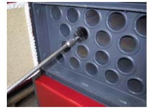
Cleaning the tubes
