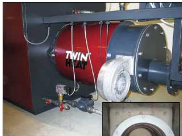
The combustion of the biofuel takes place in the water-cooled burner. The combustion air in the burner is heated to 300–400°C.
