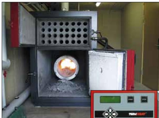
The large door of the boiler provides good access during inspections of boiler/burner. The top door provides access to the heat exchanger of the boiler where the flue gasses are cooled.
