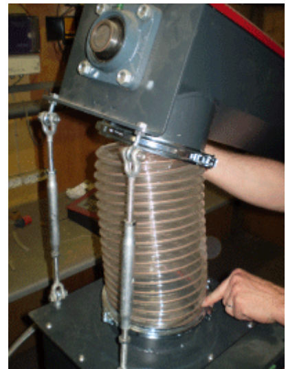
Stay tighteners mounted between auger and rotating valve on boiler
